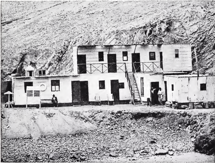
HEADQUARTERS OF THE COMPAÑIA ADMINISTRADORA DEL GUANO, ON THE SHORE OF THE SOUTH STRAIT, CENTRAL CHINCHA ISLAND
